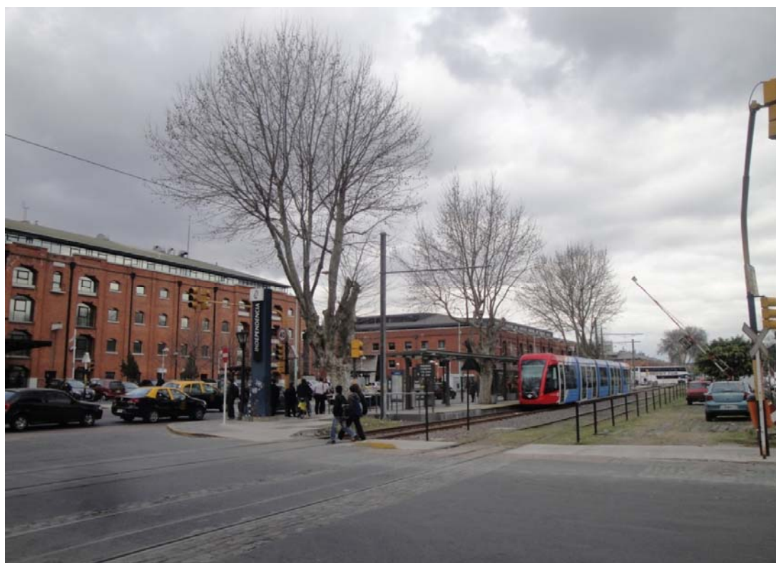
Figure 1. New tram line in Puerto Madero, Buenos Aires
