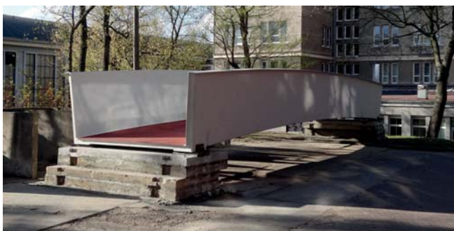
Fig. 2. Footbridge built on the Gdansk University of Technology campus territory within the framework of the project FOBRIDGE
