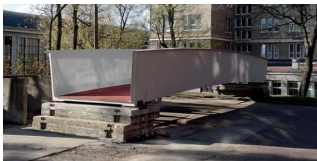
Fig. 2. Footbridge built on the Gdansk University of Technology campus territory within the framework of the project FOBRIDGE
