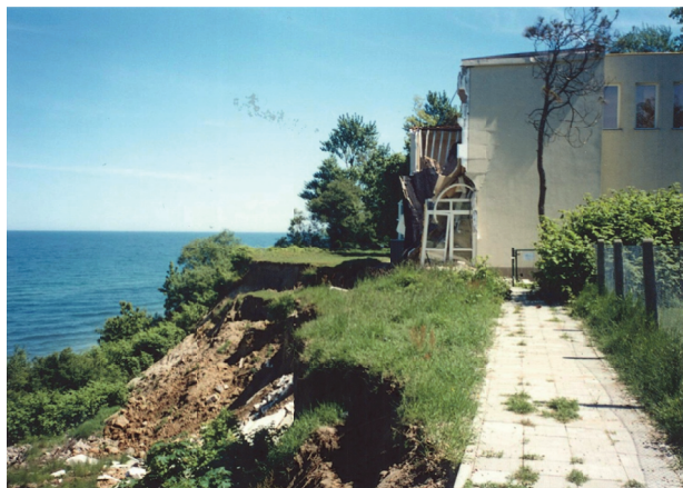
Fig. 2. The leisure centre "Horyzont" situated on the edge of an active cliff and damaged in 2002. (photo courtesy of W. Subotowicz)
