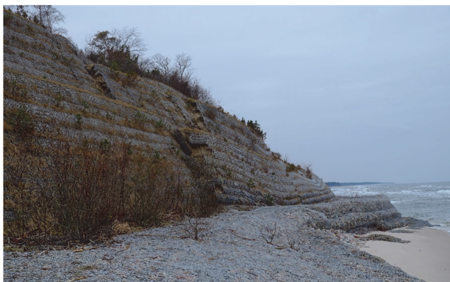
Fig.4. Degradation of reinforced cliff part at Jastrzebia Gora – situation of January 2017.
