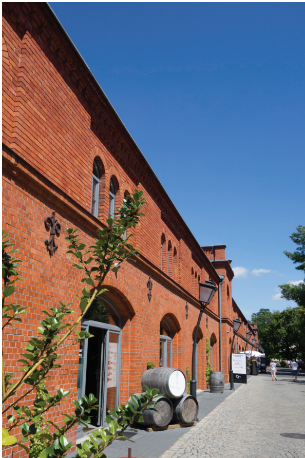
Figure 7. Poznań (Poland), City Park – shops and restaurants in the historical military buildings. Source: photo E. Raszeja
