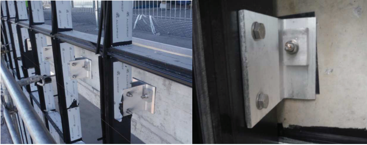
Fig. 1. Mullion-transom wall system – aluminium profiles and brackets
