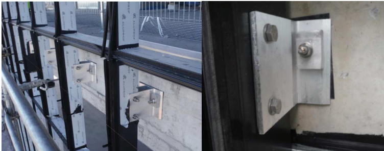
Fig. 1. Mullion-transom wall system – aluminium profiles and brackets
