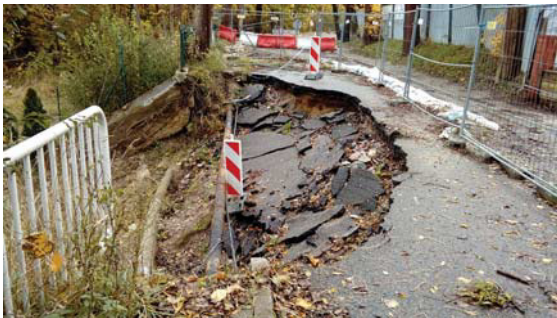
Fig. 4. A cavern and hydraulic piping flow canal revealed after the damage [10]
