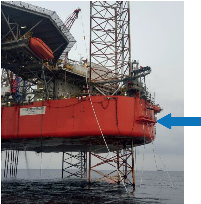
Fig. 12. Risers mounted on LOTOS Petrobaltic platform, along with CTP injection pipes
