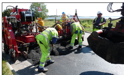
Figure 8: Construction of the first Danish full scale test track in Kalvehave (Kalvehave I): the fresh PERS mix in front of the gussasphalt paver was first spread manually (left hand side) and then compacted (right hand side)
