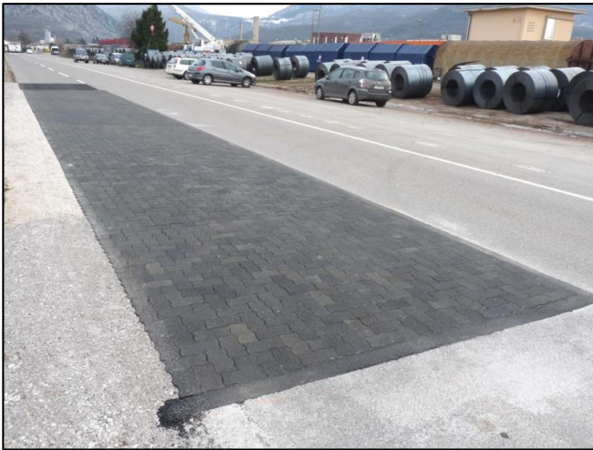
Figure 15: Just finished Slovenian full scale test track in Nova Gorica (Picture: D. Kokot)
