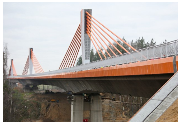
Fig. 1. Side view of MS-3/DK-16 bridge.
