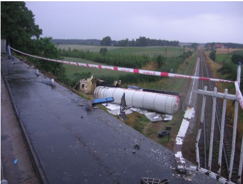
Fig. 1. Fall from the viaduct of the car - a cistern with 20t of propane-butane gas (source: Provincial Police Headquarters - Gdańsk).
