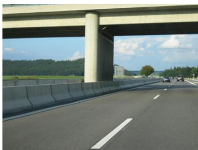
Fig. 1. Concrete barrier protecting the bridge column (source: www.debonte.com ).
