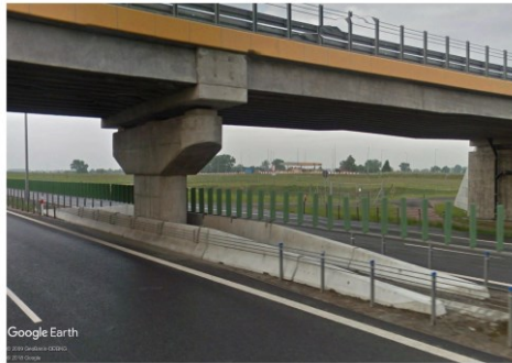
Fig. 1. Bridge column protected by concrete road safety system, credits: Google Earth.
