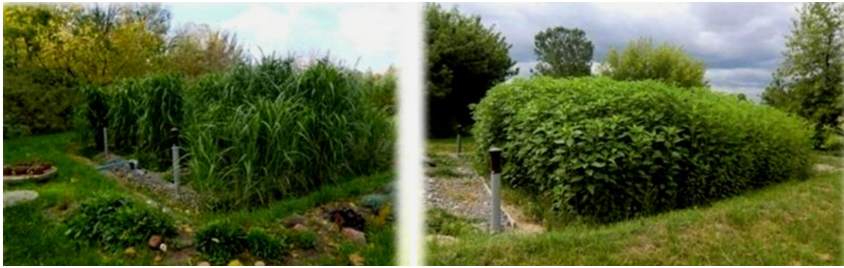
132 133 Photo 1. Hybrid constructed wetland, VF-HF type, with giant miscanthus (on the left) and 134 Jerusalem artichoke (on the right) (Józwiakowski, 2016) 135
