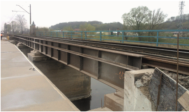
Fig. 1. Bridge over Radunia River in Gdańsk (Poland)
