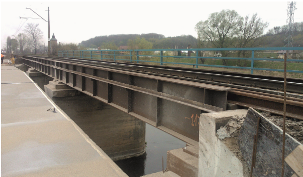
Fig. 1. Bridge over Radunia River in Gdańsk (Poland)
