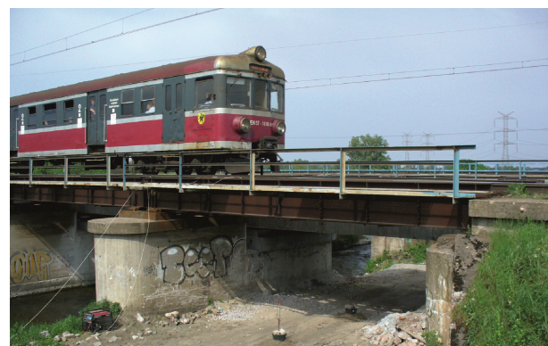
Fig. 4. Field measurements – the bridge under EN57 train
