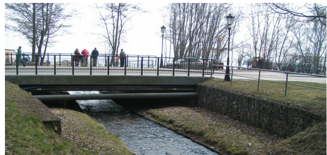
Fig. 4. The bridge over Kacza river in line of Orłowska street in Gdynia (a photo from this author's archive),
