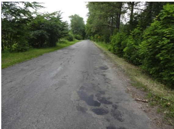
Fig. 2 – Example of a provincial road pavement qualified for cold recycling.
