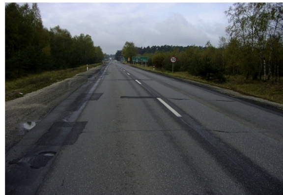
Fig. 1 – Example of a national road pavement qualified for cold recycling.
