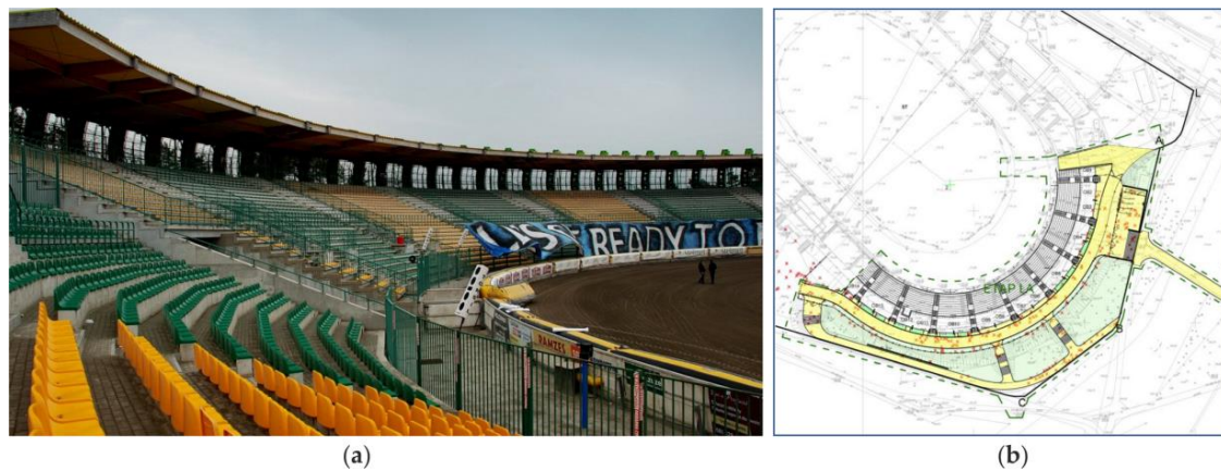
Figure 2. Swiss Krono Arena: (a) the view on the grandstand, (b) the location of the grandstand on the land development plan.
