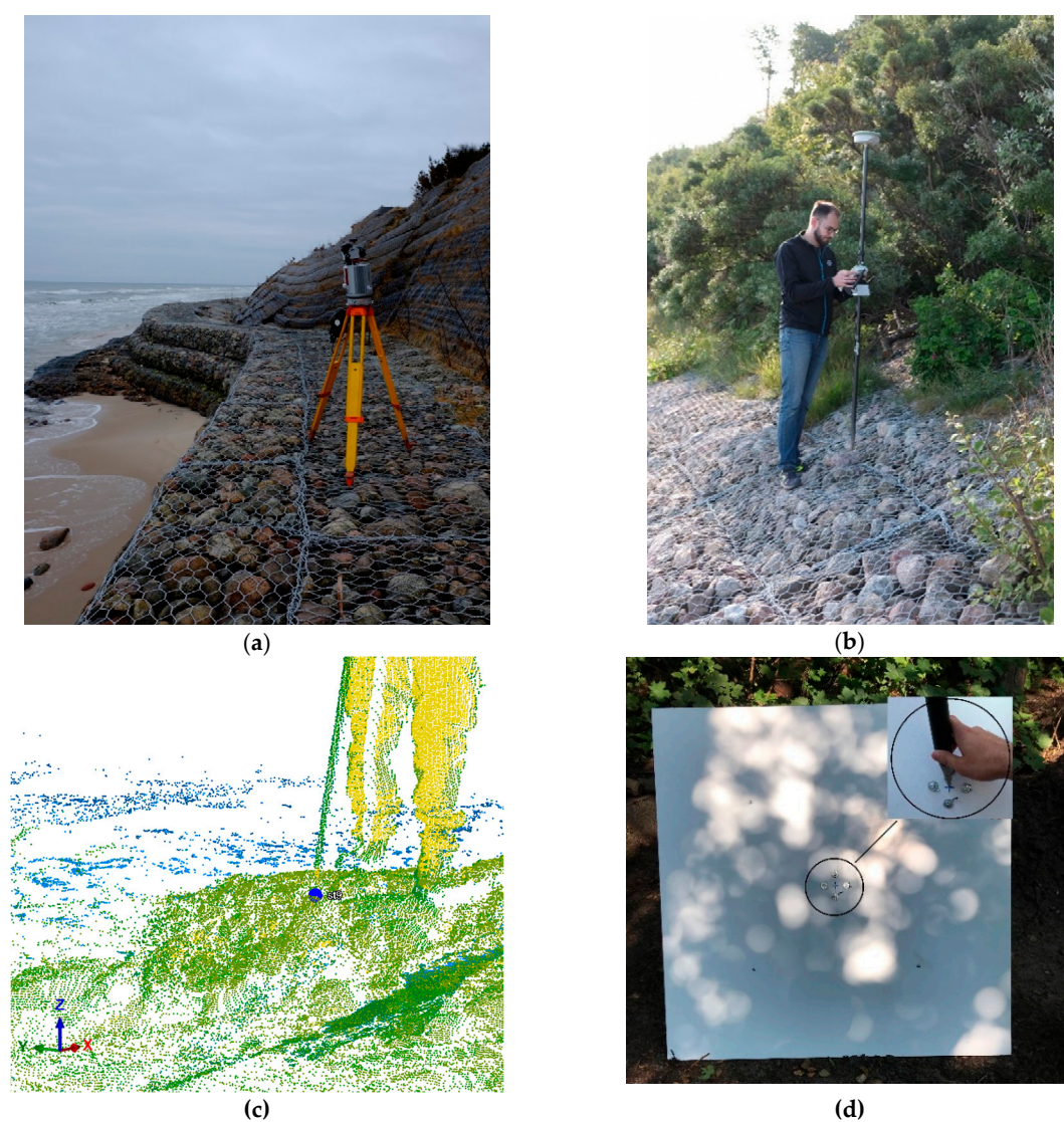
Figure 4. (a) The laser scanner working on the investigated object; (b) the Global Navigation Satellite System (GNSS) receiver; (c) the point cloud with the marked bottom of the pole; and (d) the materialized tie point z with a marked sighting cross on which we put a pole.
