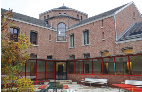
Fig. 9. Former in Prison in Hasselt, exterior (photo by J. Szczepański)
