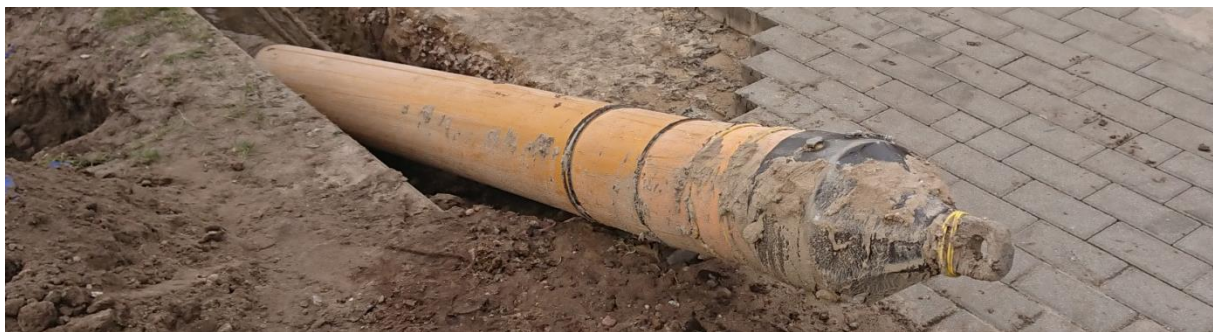
Figure 14. Leading the pipe in the entrance chamber
