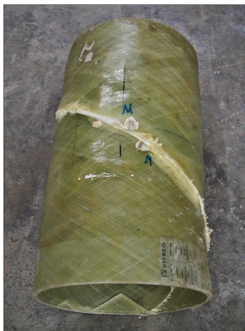
Fig. 9. Destroyed composite coating
