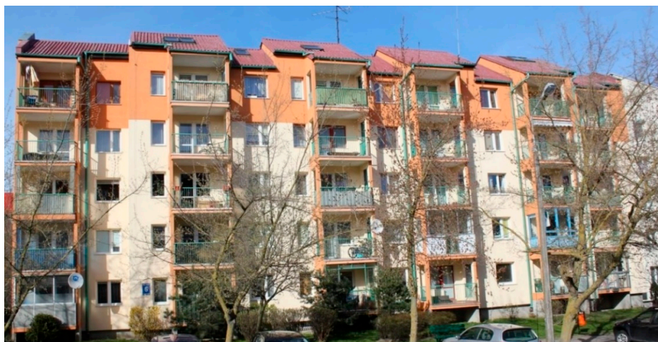
Figure 3. A multi-family, five-story, three-frame residential building. Source: own photo of the authors.
