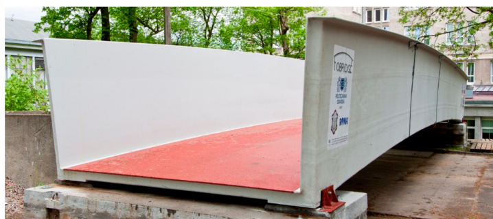
Figure 1. Composite footbridge designed within the FOBRIDGE project.
