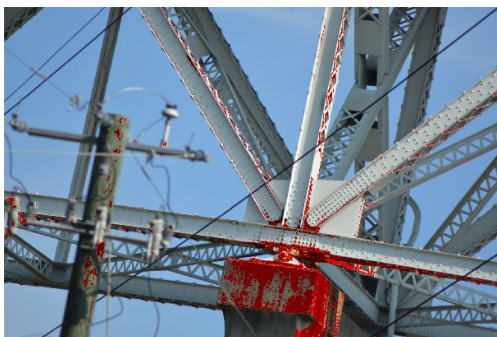
Figure 15. A database of rust colour pixels.
