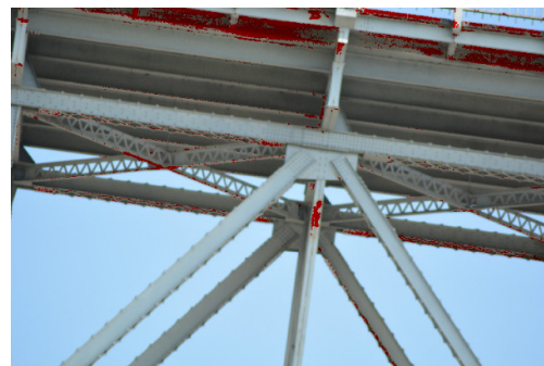
Figure 15. A database of rust colour pixels.
