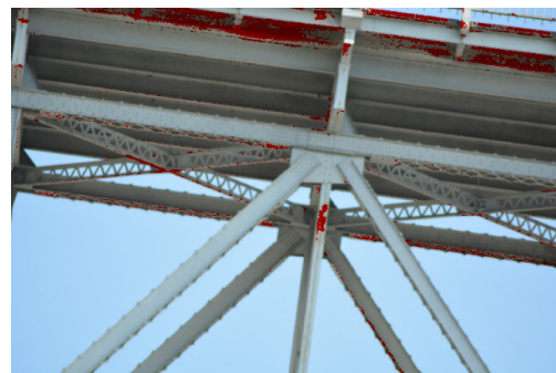
Figure 15. A database of rust colour pixels.
