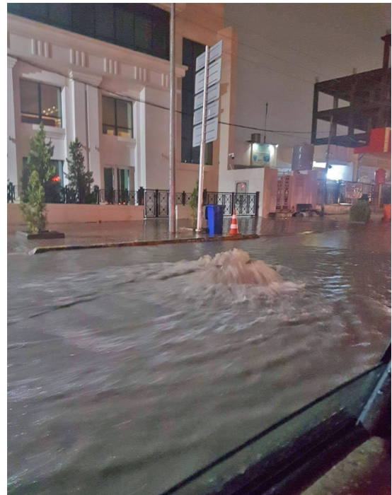
Fig. 11a. Overflow occurring in one of the man-holes on a street in Erbil
