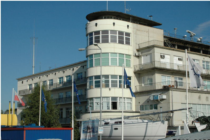
Fig. 3 Former Polish Sailor's House, now the Navigation Faculty of the Maritime Academy in Gdynia, designed by Bohdan Damiński and Tadeusz Siczkowski in 1937, started in 1938-1939 and completed after 1945 (photo: M. J. Sołtysik)
