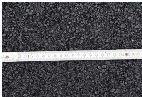
Figure 12. Finished texture of the poroelastic wearing course.
