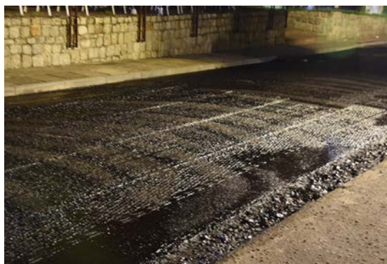
Figure 9. Milled surface of the binder course.
