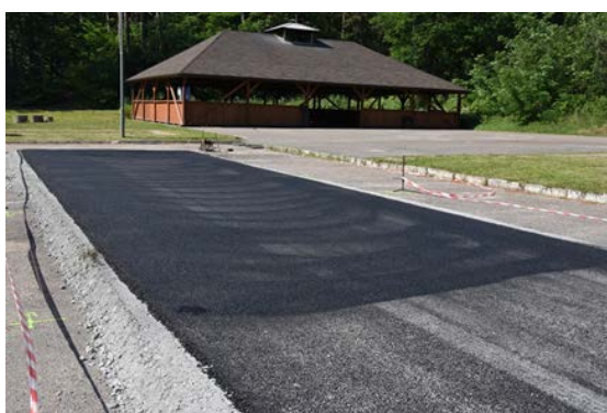
Figure 14. Binder course AC 16W before installation of different types of wearing courses.
