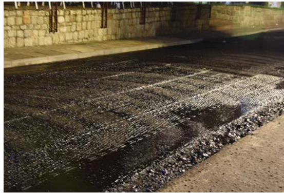
Figure 9. Milled surface of the binder course.
