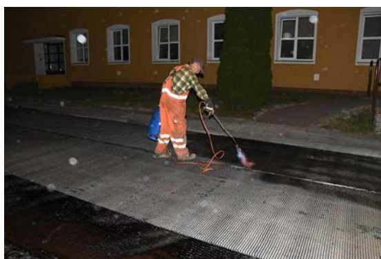
Figure 10. Applying glass geogrid on the surface of the binder course.
