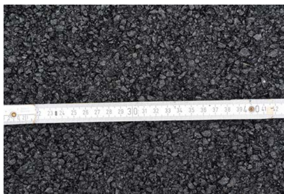
Figure 12. Finished texture of the poroelastic wearing course.
