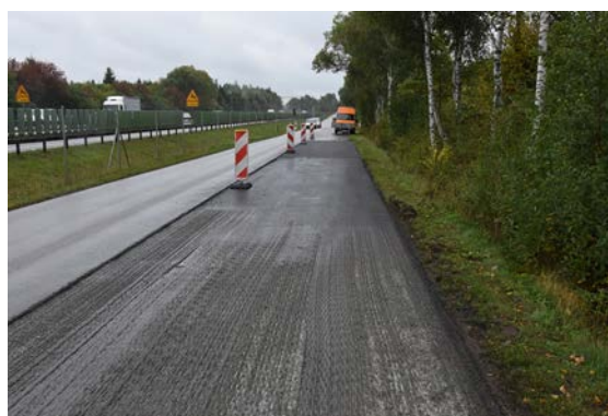
Figure 17. New binder course after surface milling.
