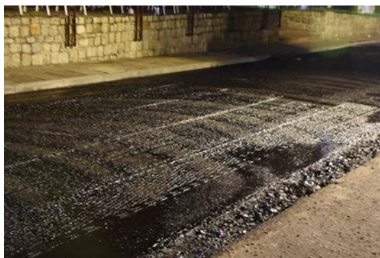
Figure 9. Milled surface of the binder course.
