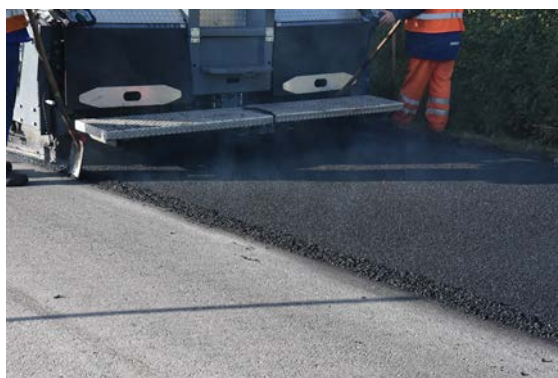
Figure 18. Laying of the poroelastic mixture.
