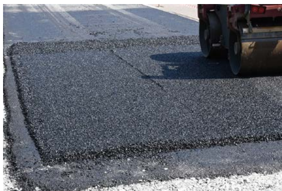
Figure 15. Compacting of PA 11 mixture.
