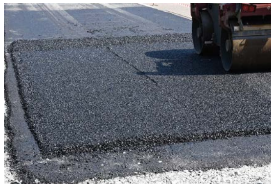
Figure 15. Compacting of PA 11 mixture.
