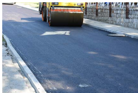
Figure 8. Compaction of the binder course AC 16W.
