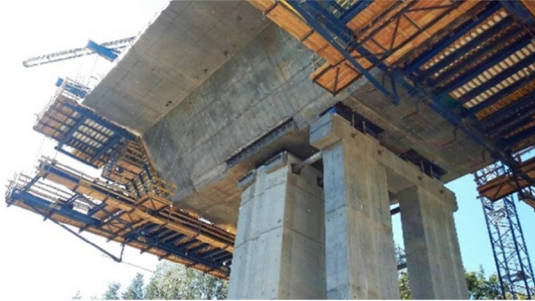
Fig. 10. Monitored section no. 4.4.
