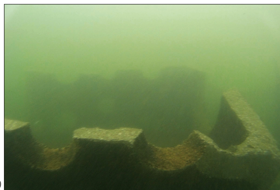
Fig. 9. Damaged elements under water
