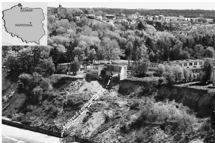
Fig. 1 A general view of the cliff in Jastrzębia Góra. The aftermath of the 2002 landslide for adjacent buildings is clearly visible
