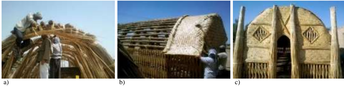
Fig. 10a, 10b, 10c: Construction processes of Mazif
