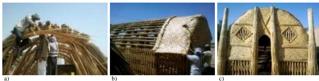
Fig. 10a, 10b, 10c: Construction processes of Mazif
