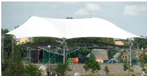
Fig. 1. Membrane hanging roof in Pruszcz Gdanski
