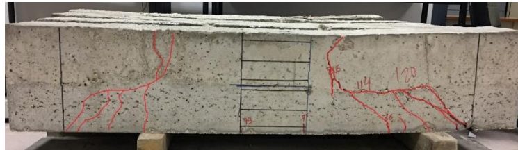
Fig.11: Beam (B3) at failure
