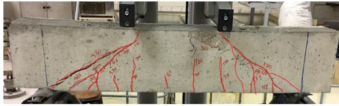
Fig.9: Beam (B1) at failure
