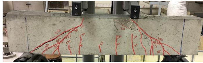
Fig.9: Beam (B1) at failure
