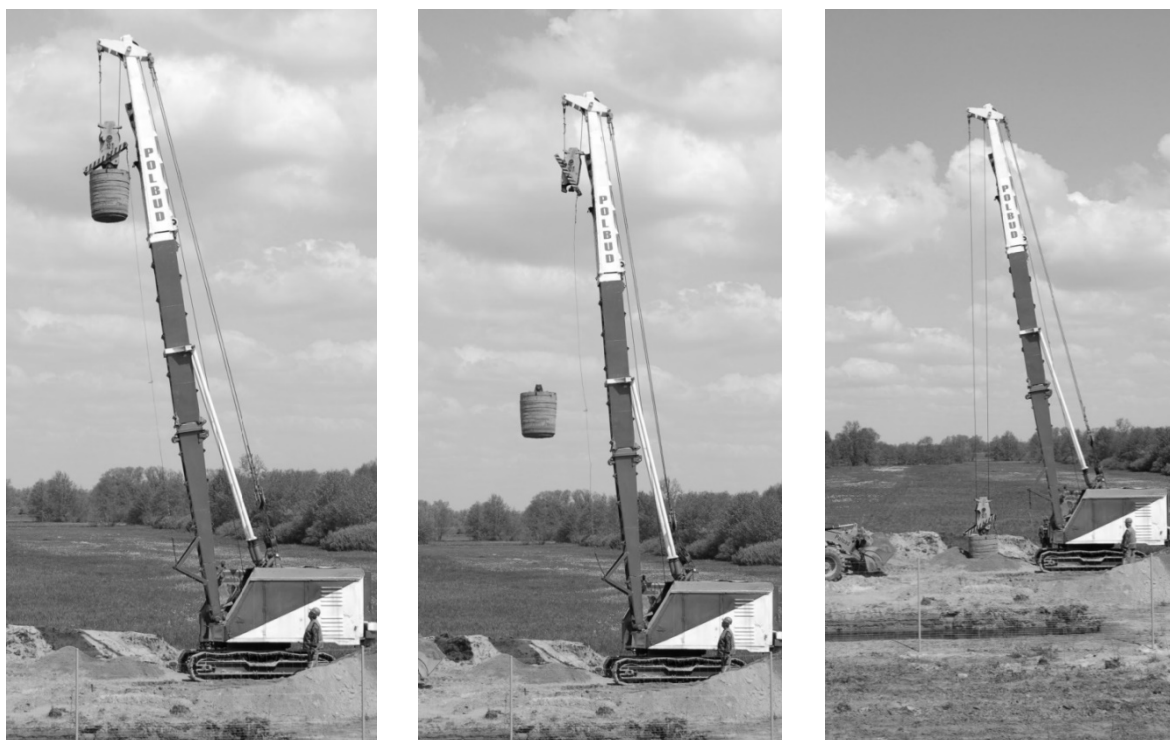
Figure 7. Dynamic replacement in practice.
