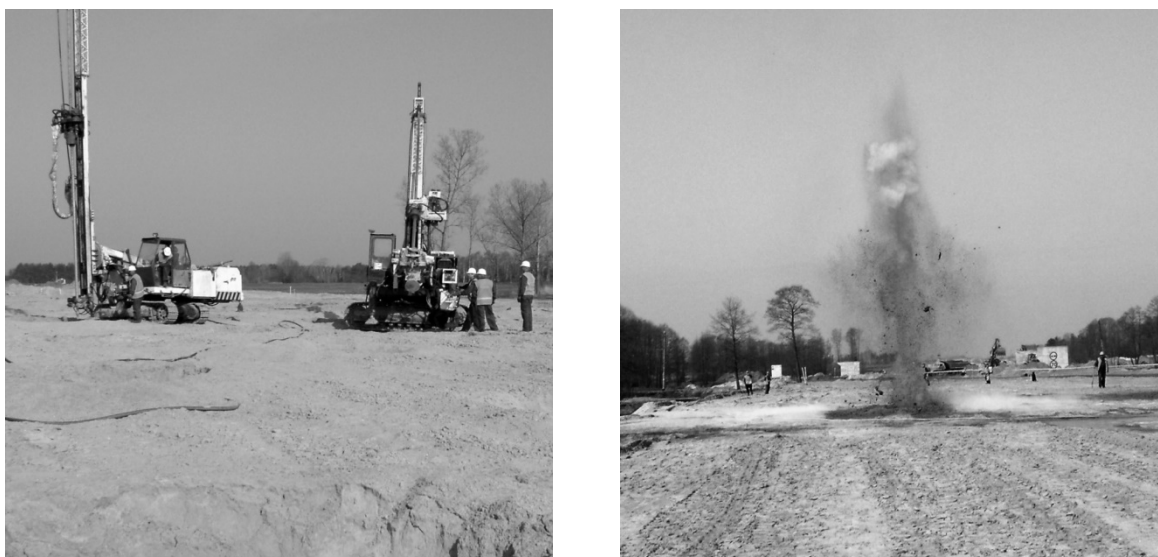
Figure 6. Blasting charge in practice.
