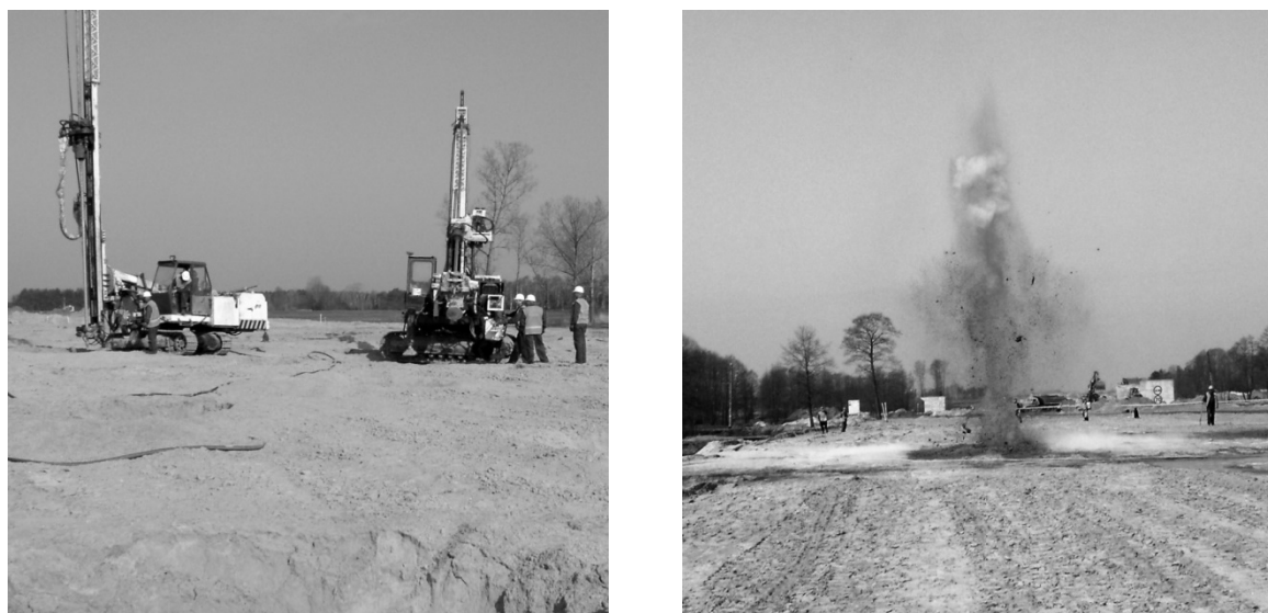
Figure 6. Blasting charge in practice.
