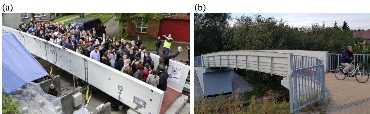
Fig. 1. The footbridge (a) during examination in Gdansk University of Technology campus [46], (b) installed for public traffic over Radunia River near Gdańsk, Poland
