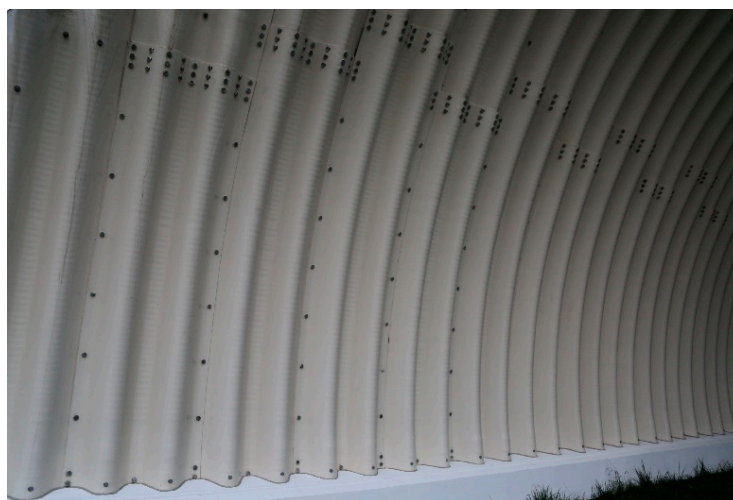
Figure 3. The corrugated steel sheets and their bolt connections.
