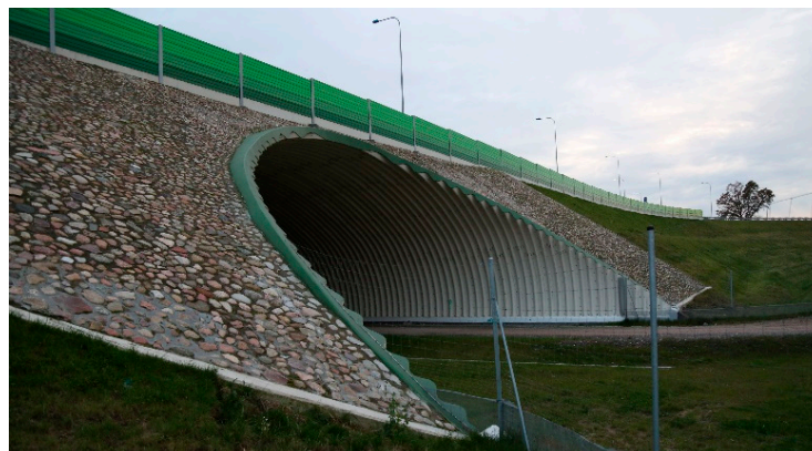
Figure 2. Close up of one of the bridge sides taken in October 2019.
