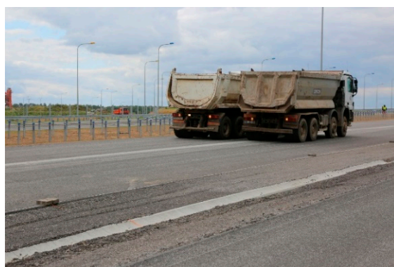
Figure 12. The trucks moving between M23 and M24 testing positions.
