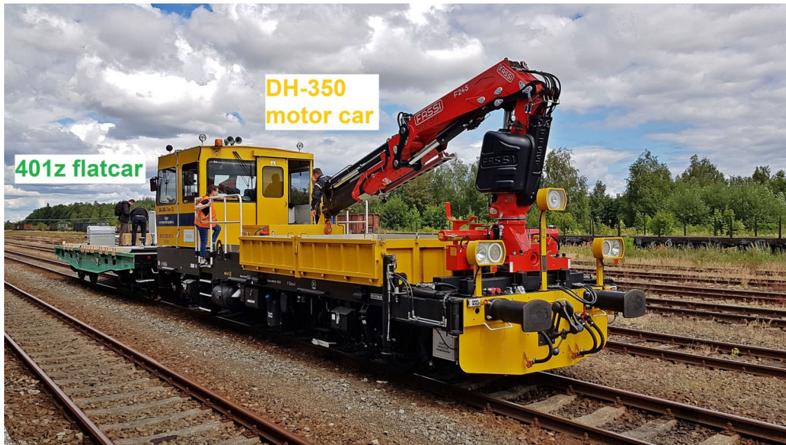
Figure 5. Measuring set number 3 for making mobile satellite measurements.
