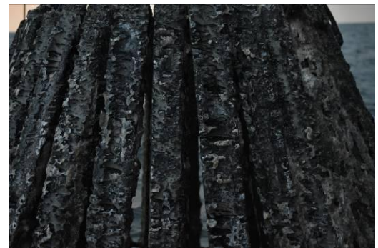
Photos 4–9. One of the cone-shaped anodes basket during a cleaning procedure carried out at sea. The upper three photos show the cone before hydro-cleaning, and the lower three photos show the cone after is cleaned.
