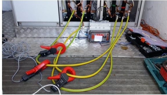
Figure 10. Sheaths unearthed and uncrossed in Substation 2.
