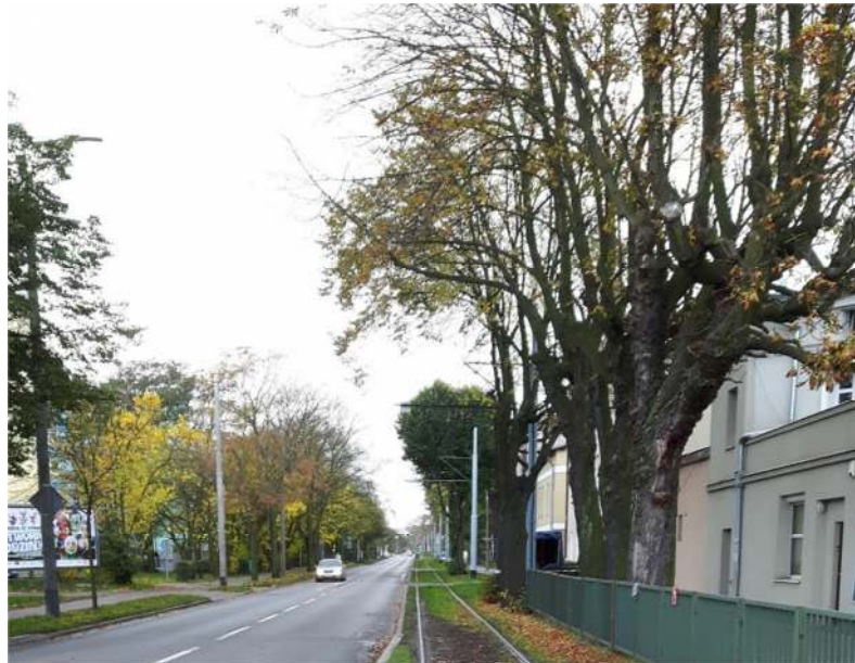
4. The condition of the track and terrain obstacles along the section c
