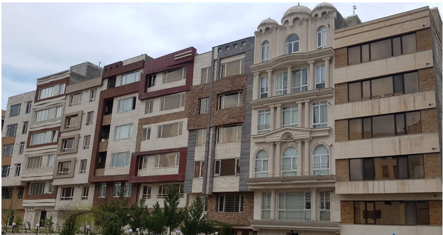
Fig. 1 Adjacent buildings in Tehran with different floors and base levels without separation distance
