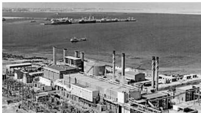
Fig. 2. Ras Abu Aboud Power Station in early Years
