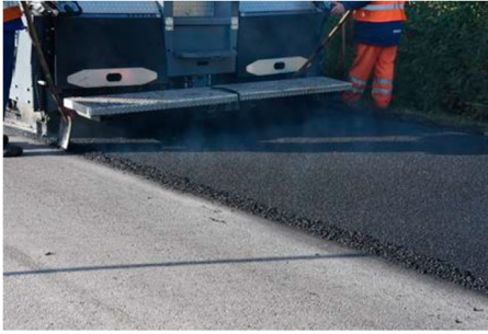
Figure 13. (A) Laying of the poroelastic mixture; (B) close-up view of the poroelastic wearing course.
