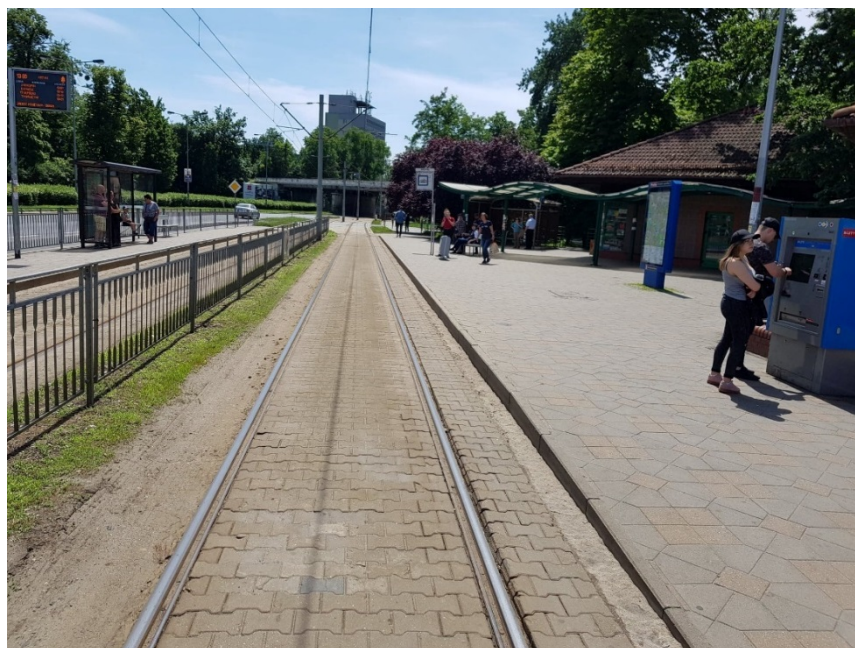
Fig. 6. Tram platform stops located in Krzyki tram loop in Wrocław (Poland)
