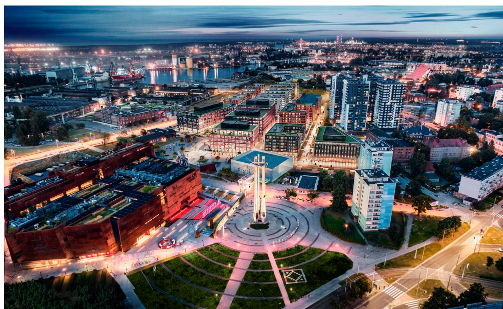
Figure 13. The construction of the DOKI investment became possible after the demolition of some barracks. The project scale is large. The new development is going to infill the area between the ECS (bottom left), the Bastion Wałowa (very densely erected four towers on the upper right—
