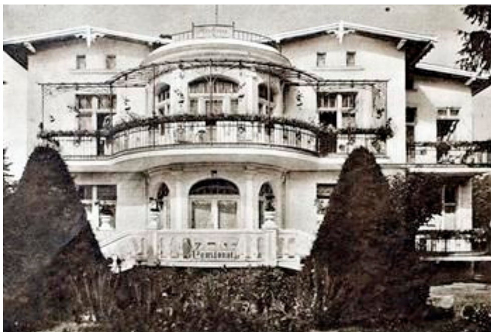
Figure 6. Willa Halina seen from the front. Photo from 1934. Source: http://www.dawnysopot.pl/index.php?content=przewodnikopis&obiekt=willahalina . (accessed on 29 April 2021).
