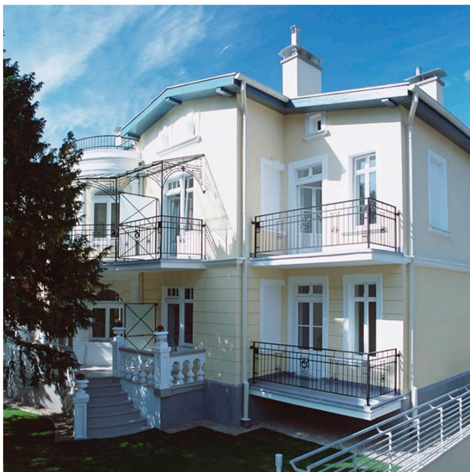
Figure 13. Historical part of Willa Halina. Front elevation after revitalization. Source: FORT Taraszkiewicz Architekci.
