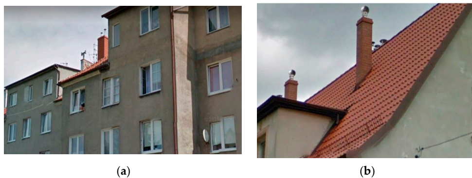
Figure 21. Multi-family housing in Gdańsk: (a) traditional chimney cap and (b) rotary type chimney cap.
