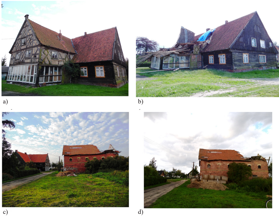
Fig. 3. Destruction of the arcaded house in Izbiska: a) August 2016, b) June 2017, c) view of the farm – August 2016, d) view of the farm – September 2020 ( photo by the author )
