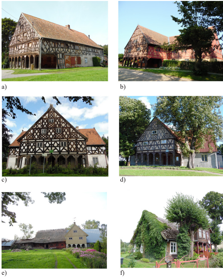
Fig. 1. Types of arcaded houses: a) type I house in Klecie, b) type II house in Trutnowy, c) type II-III house in Stalewo no.14, d) type III house in Koszwały, e) type III house in Markusy, f) type III house in Mikoszewo no. 68 (photo by the author)
