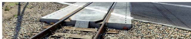
Fig. 8. Concrete level crossing slabs
